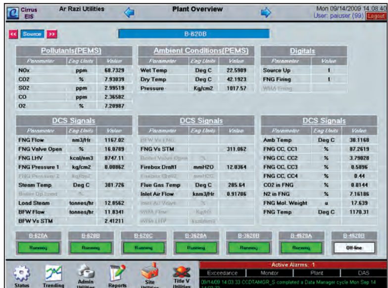
FIGURE 5. This typical DAS reporting screen shows the status of all input parameters for one of the seven boilers. The green boxes at the bottom of the screen show that six of the seven boilers are running and one is shut down
